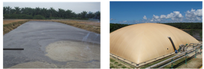
Figure 1: POME and a covered lagoon digester
